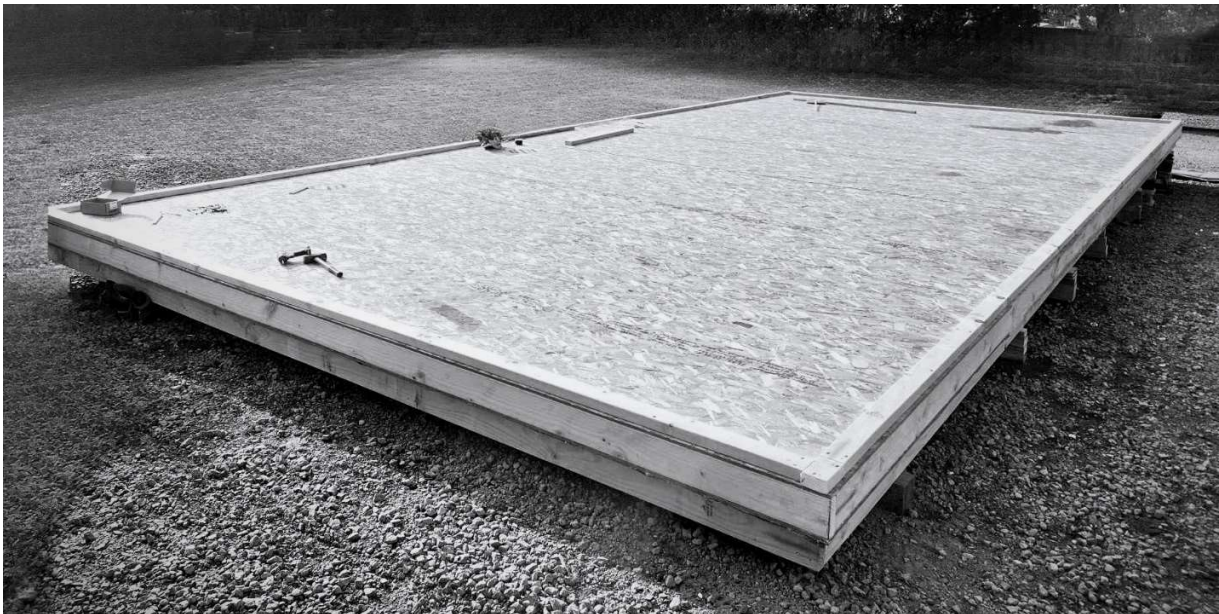
Figure 3: Floor panels installed on subfloor bearers
