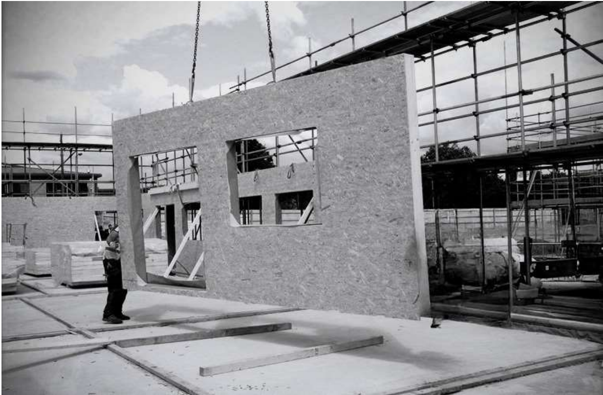
Figure 8: Big format panel being craned into place
