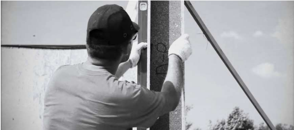
Figure 6: Panel being set plumb and level prior to fixing to bottom plate
