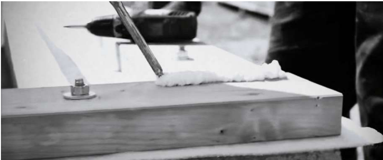
Figure 4: Timber bottom plate installed on concrete floor
