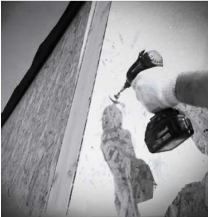
Figure 7: Corner panels being connected with SIP screws
