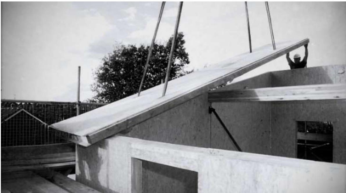
Figure 2: Roof panel being lifted into position
