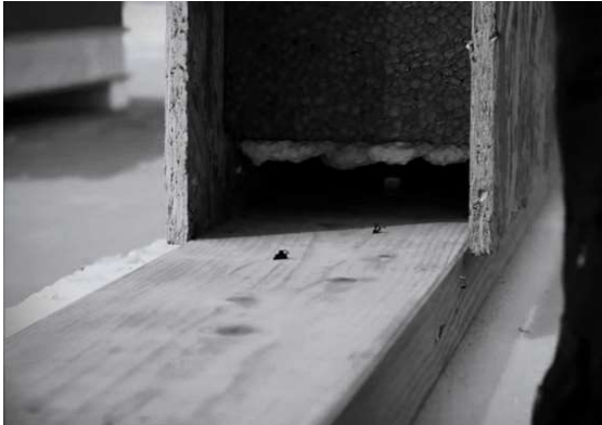
Figure 9: Panel with expanding foam being fitted to bottom plate
