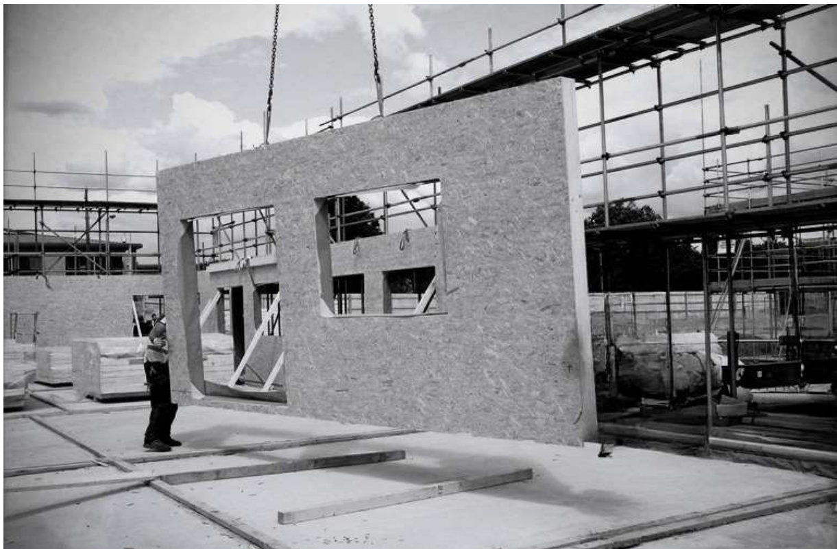
Figure 1: Wall panel being lifted into position
